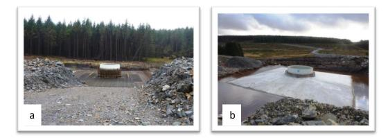
Figure 52. Turbine base installation at Arecleoch showing the rebar (left) and concrete surround (right). Both illustrate the extent of peat removal and disturbance potential and in the image on the right the excavation has filled with DOC rich water.
